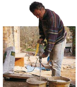
el albañil construction worker
